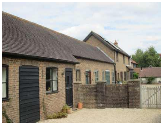
Fig.14: Example of Local Housing
