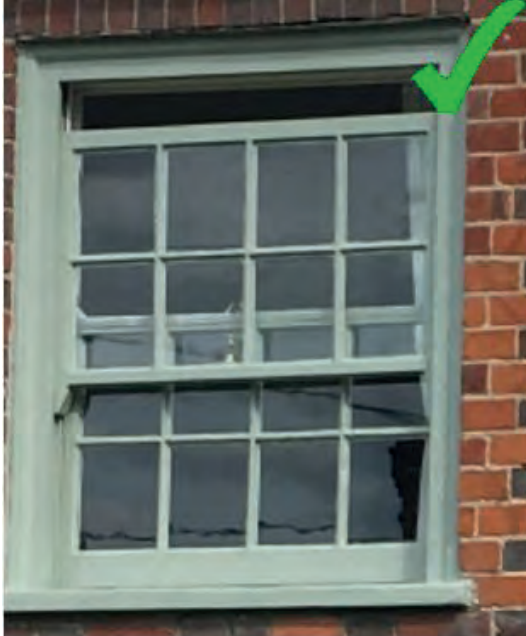
Photograph of a window with historic glass which creates a distinctive reflection and distortion
