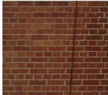
English bond with alternate rows of headers and stretchers
