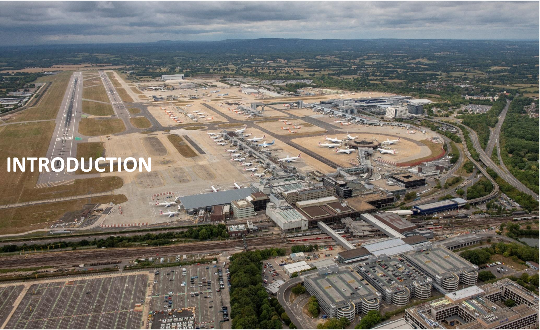
Aerial view of Gatwick Airport with the South Terminal and Gatwick Railway Station in the foreground
