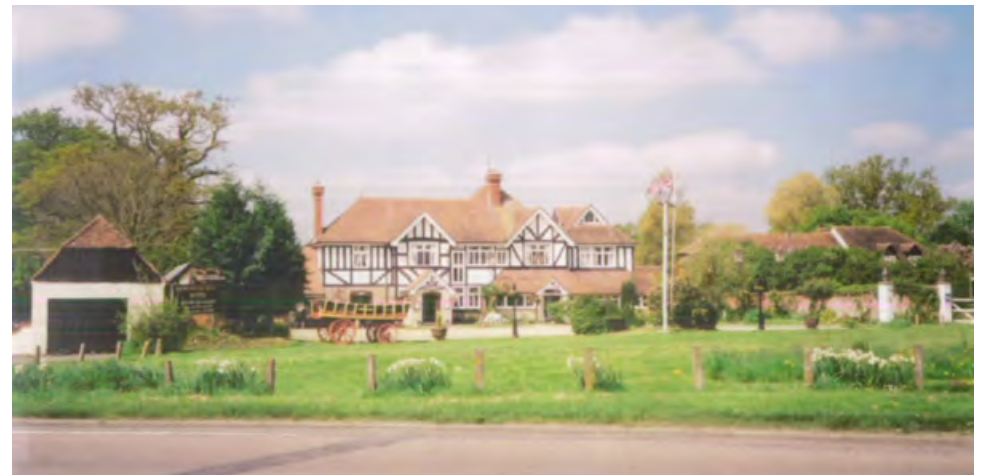
Photograph of Newstead Hall Hotel prior to demolition (sourced from planning history)
