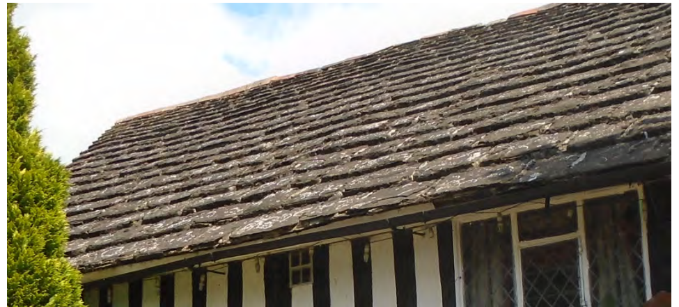
Horsham Stone slate roof
